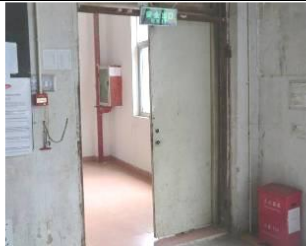
Exit and fire alarm
